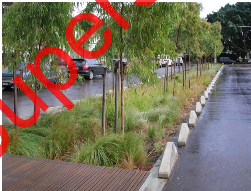
Plate 3-3: Median Strip Bioretention applications
