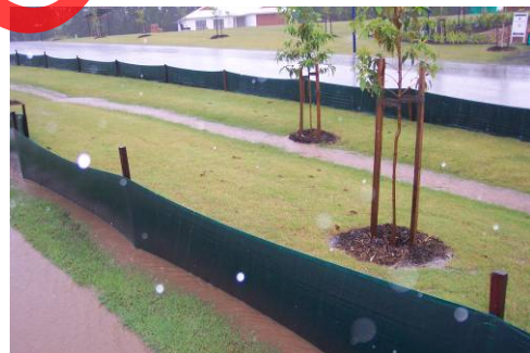
Plate 3-6: Bioretention Swale Sediment & Erosion Control
