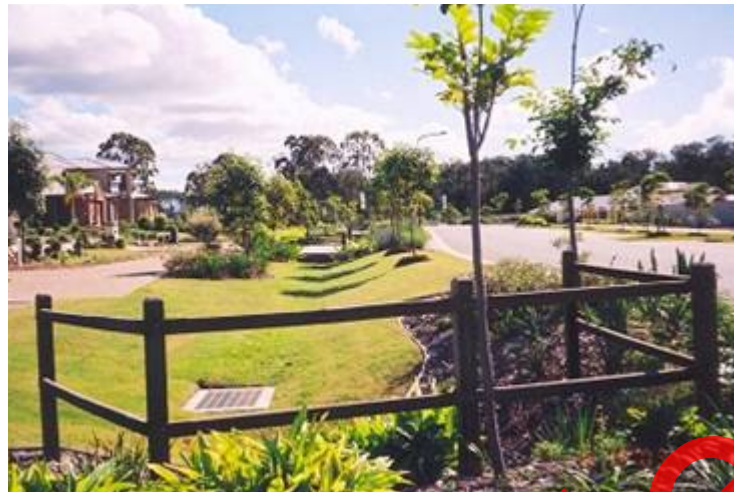
Plate 3-7: Bioretention Swale Located Between a Main Road and Local Road
