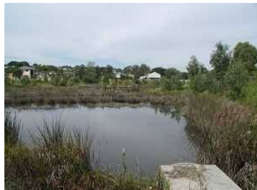
Plate 4-1: Example of Soft Edge Embankment Planting
