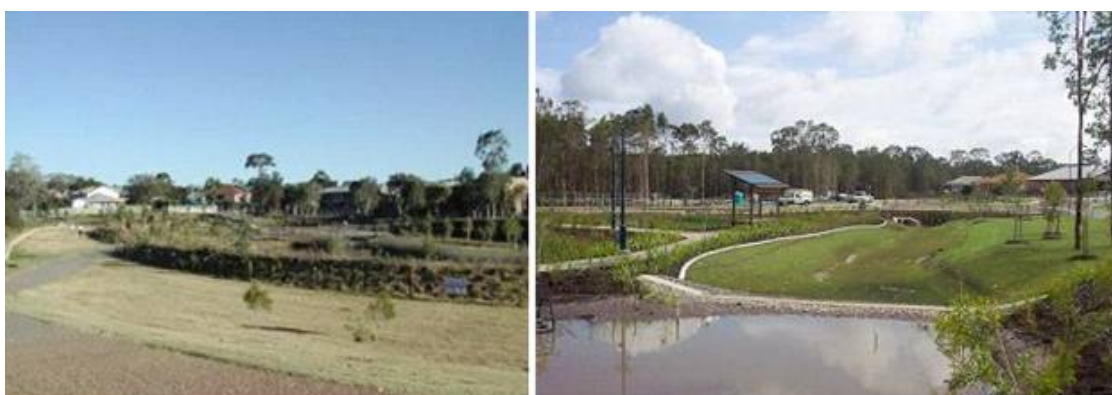
Plate 6-6: Constructed Wetland Bypass Weir and Channel Configurations
