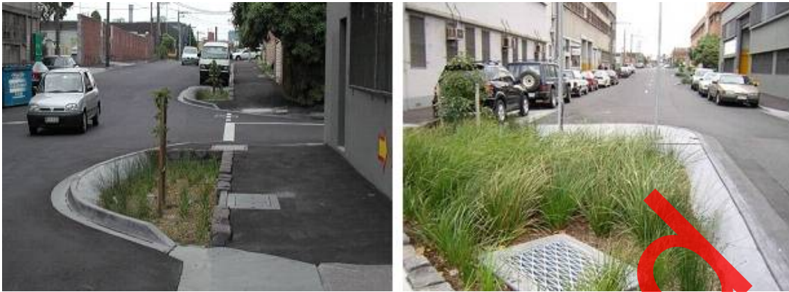
Plate 5-6: Retrofitted Bioretention System in a Street
