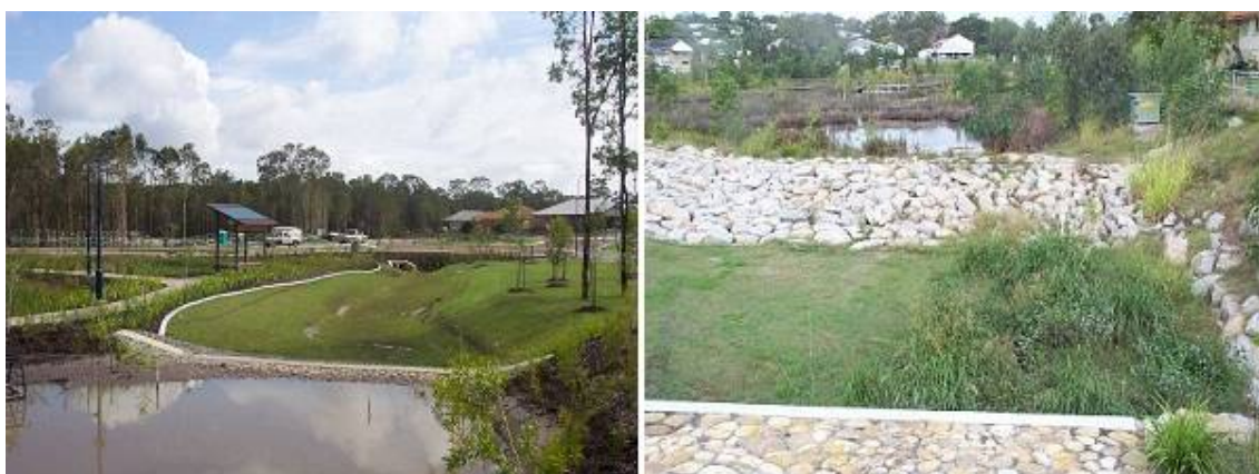
Plate 4-4: Spillway outlet weir structure of sedimentation basins at the Gold Coast and Coorparoo
