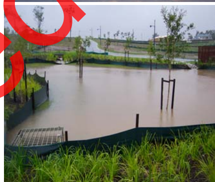
Plate 5-5 : Bioretention Basin Sediment & Erosion Control
