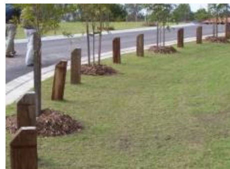
Plate 2-6: Traffic bollards mixed with street trees to protect swale from vehicles
