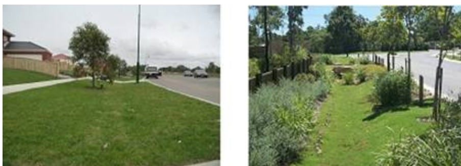
Plate 2-5: Typical sections for Swale 1 (left) and Swale 2 (right)(Note that Swale 1 also requires provision for traffic control and Swale 2 requires provision for pedestrians)
