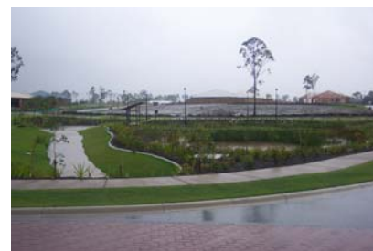
Plate 6-9: Constructed Wetland Sediment & Erosion Control Operation
