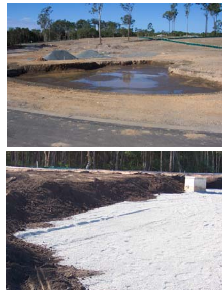
Plate 5-4: Bioretention Basin Functional Installation
