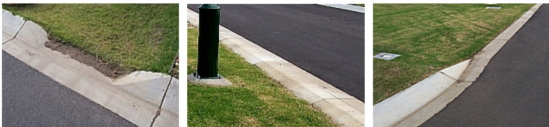
Plate 2-4: Kerb arrangements to promote distributed flow into swales
