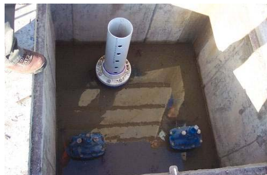
Plate 6-5: Macrophyte Zone Outlet Arrangement
