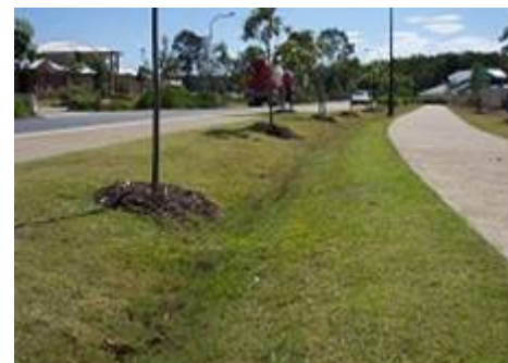
Plate 2-3: Swale incorporated into road reserve
