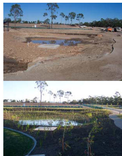
Plate 6-8: Constructed Wetland Functional Installation
