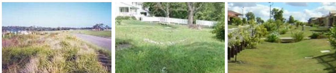
Plate 2-1: Swale systems: heavily vegetated (left), use of check dams (centre), grass swale with elevated crossings (right)
